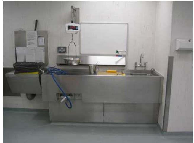
Fig. 1.21 After evisceration, the organs are often carried to a separate work area, allowing the autopsy assistant to start reconstructing the body. The work area should be well lit, with down-draft ventilation and good access to running water and drainage. All surfaces (as with other areas in the mortuary) are capable of chemical cleaning and sterilisation later
