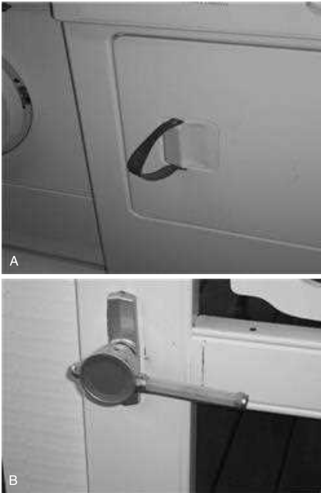
Figure 16-59 ■ Low-tech home adaptations. A , A strap is added to make a clothes dryer door accessible. B , A hole is drilled and a handle added to a screen door knob.
